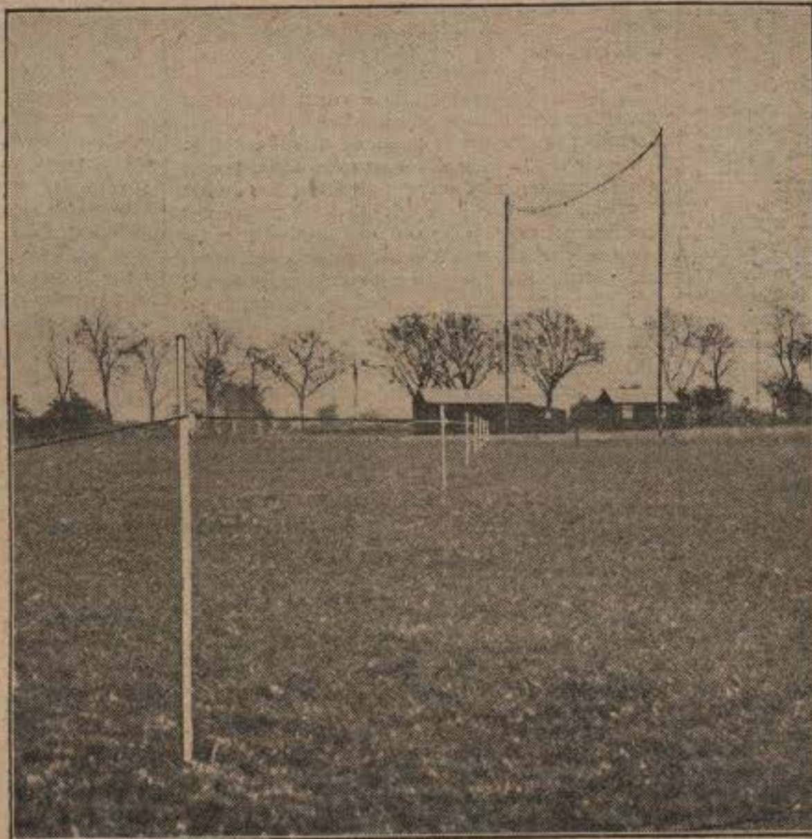
B.B.C.'S RECEIVING STATION AT KESTON.
